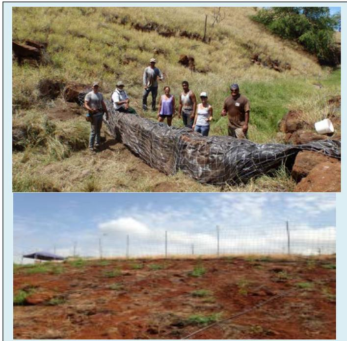
Figures 1a and b: Sediment check dams and native plants were installed to capture and reduce sediment entering the ocean.
